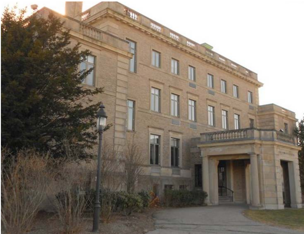
View of 2101 Commonwealth Avenue from the North
