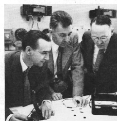
Inventors of the Bell Solar Battery, left to right, G. L. Pearson, D. M. Chapin and C. S. Fuller—checking silicon wafers on which a layer of boron less than 1/10,000 of an inch thick has been deposited. The boron forms a "p-n junction" in the silicon. Action of light on junction excites current flow.
