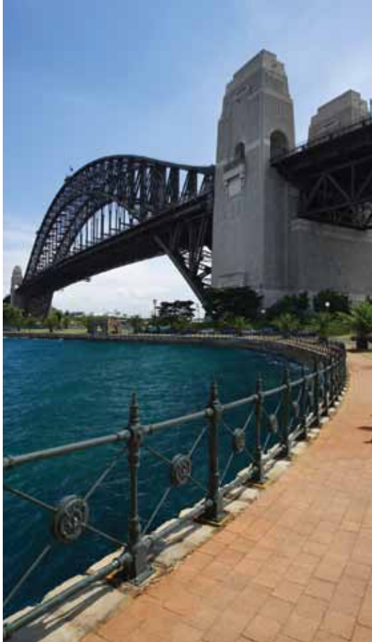
Sydney Harbor Bridge
