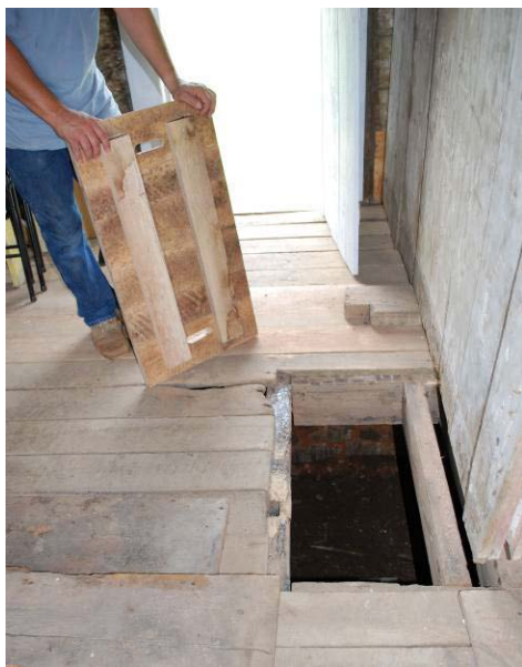
Above, Karl begins to insert his just-built cellar door that will set flush within the existing floor opening. This replaced the oversized board of plywood that haphazardly covered the entrance for many years.
